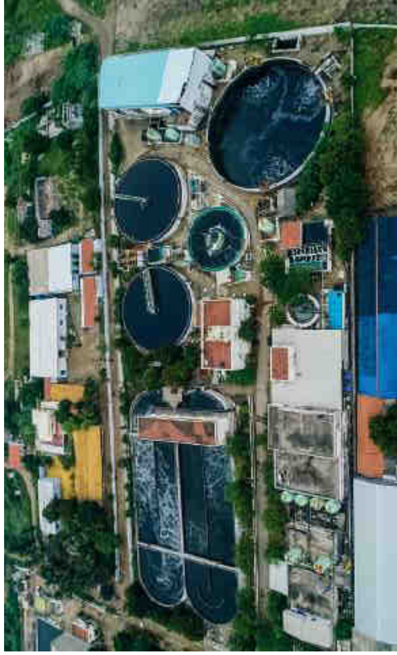
Aerial view of textile CETP at Tiruppur
