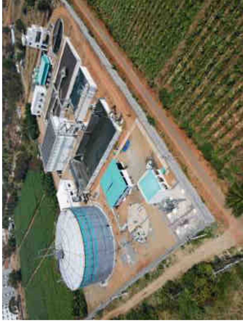
Aerial view of Sewage Treatment Plant at an Educational Institution in Erode
